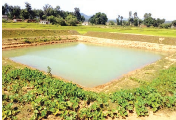
Construction of pond used for irrigation to increase agriculture yield
